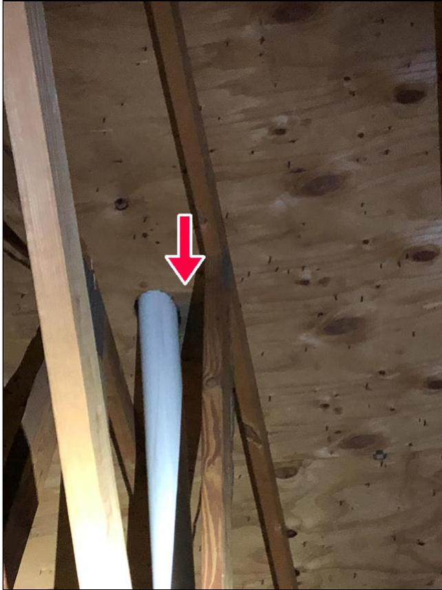
Moisture staining around vent stack
