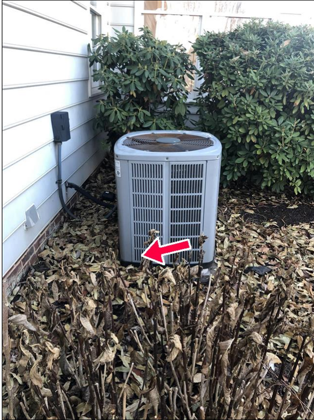
Condenser is out of level
