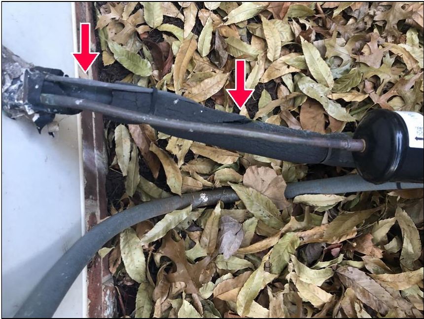
Insulation is damaged/torn
