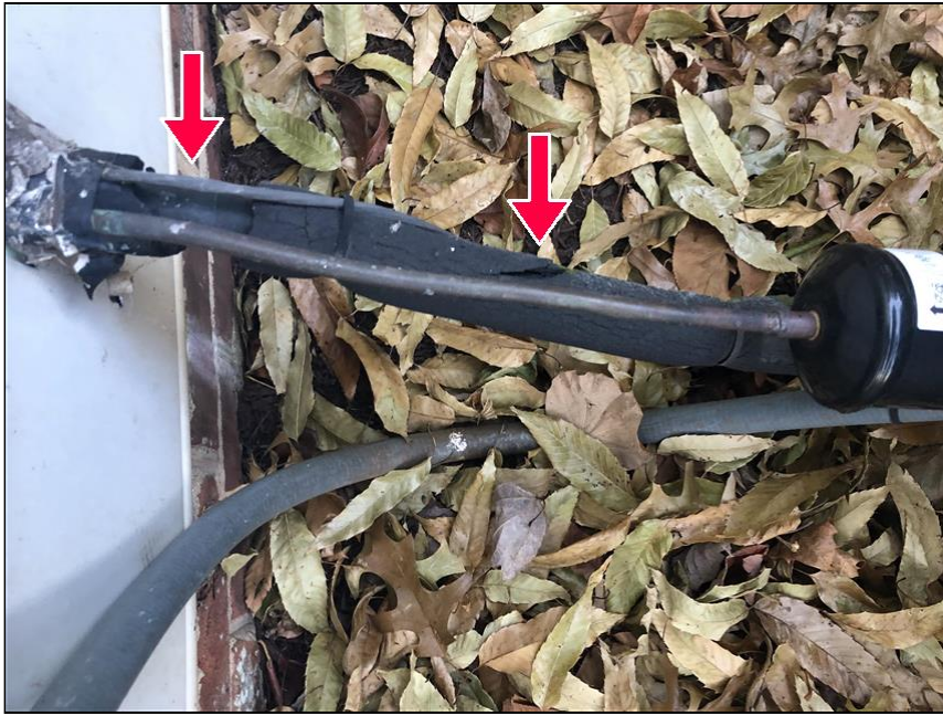
Insulation is damaged/torn
