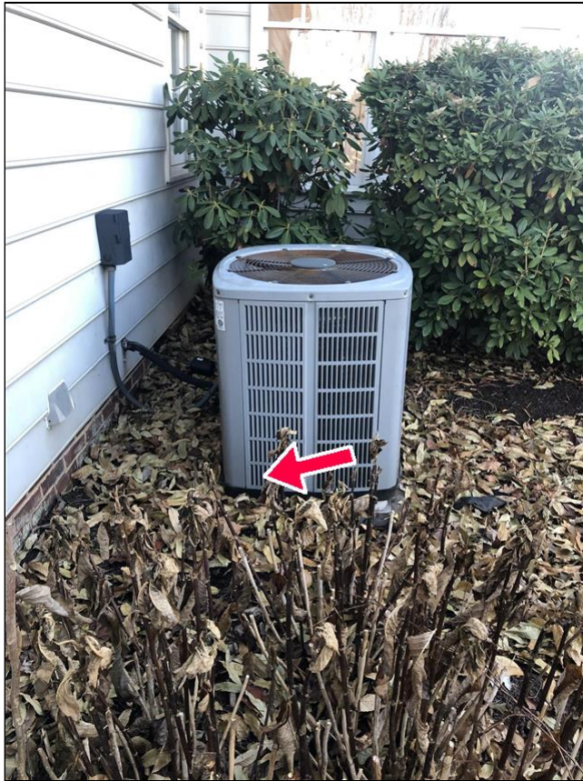
Condenser is out of level
