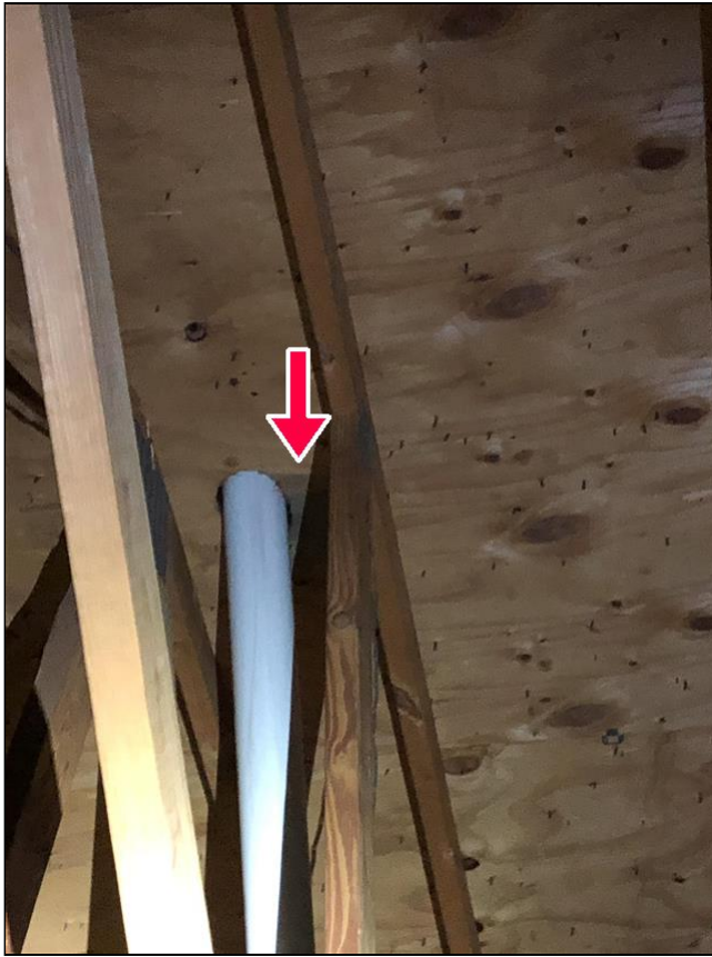
Moisture staining around vent stack
